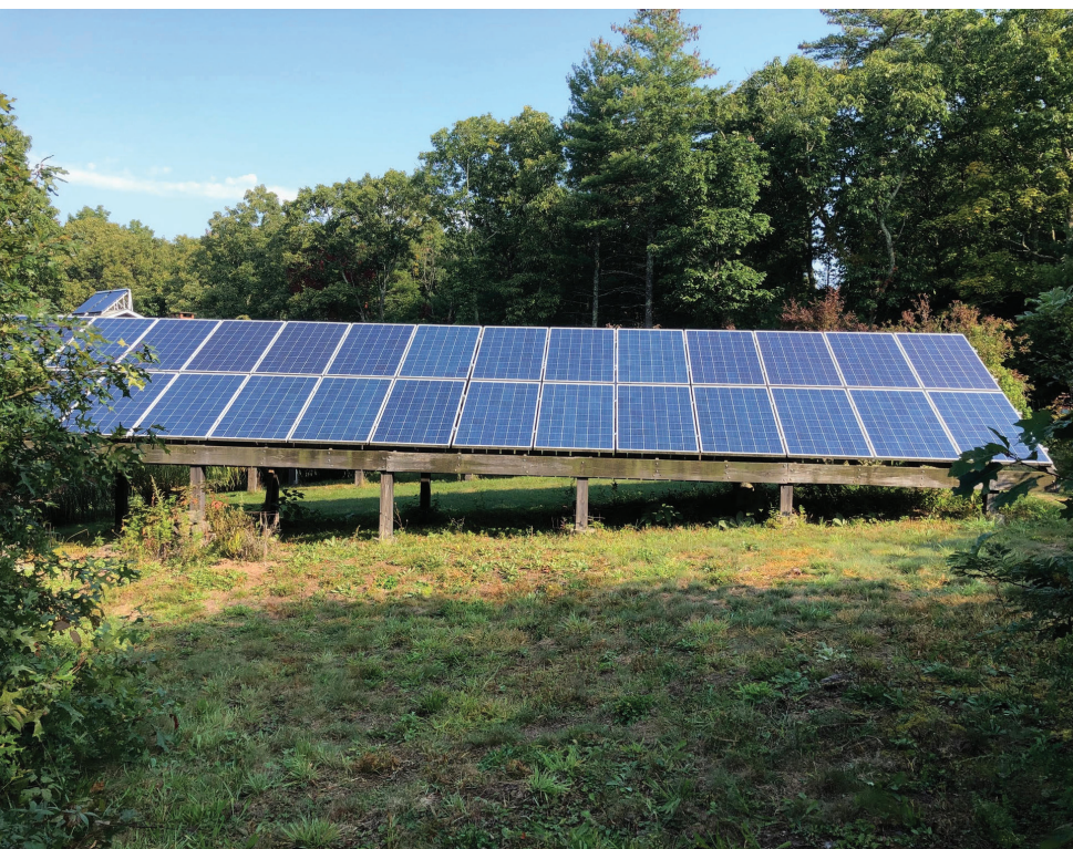
Wayne Dederick's Saugerties home with geothermal field, solar array, and electric vehicle charging station.
